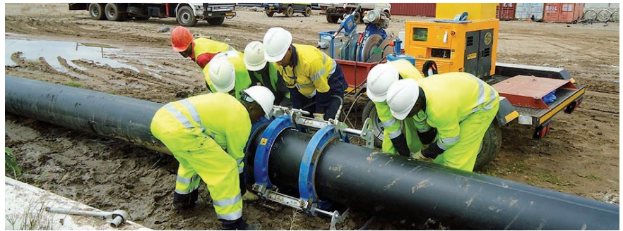
Water pipe installation and welding
