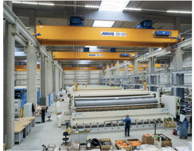
Installation at the Wiehler site
