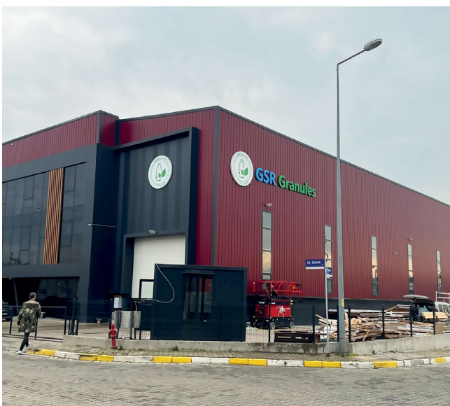
Turkish PET recycler Akmert is currently installing a Starlinger PET bottle-to-bottle recycling line at its new recycling facility in Gebze, Kocaeli, near Istanbul (Pictures ©Akmert)
