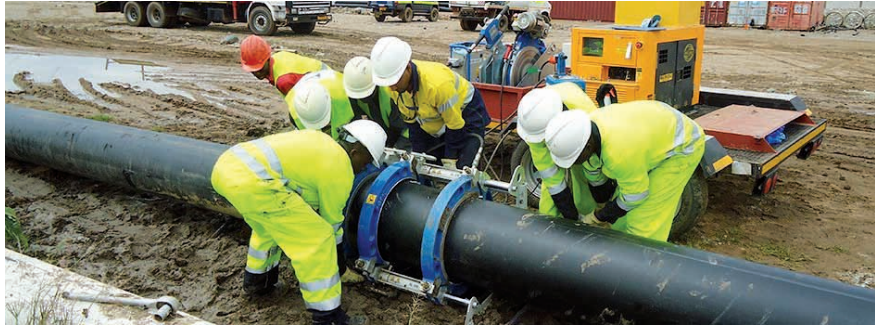
水管的安装和焊接 Water pipe installation and welding
